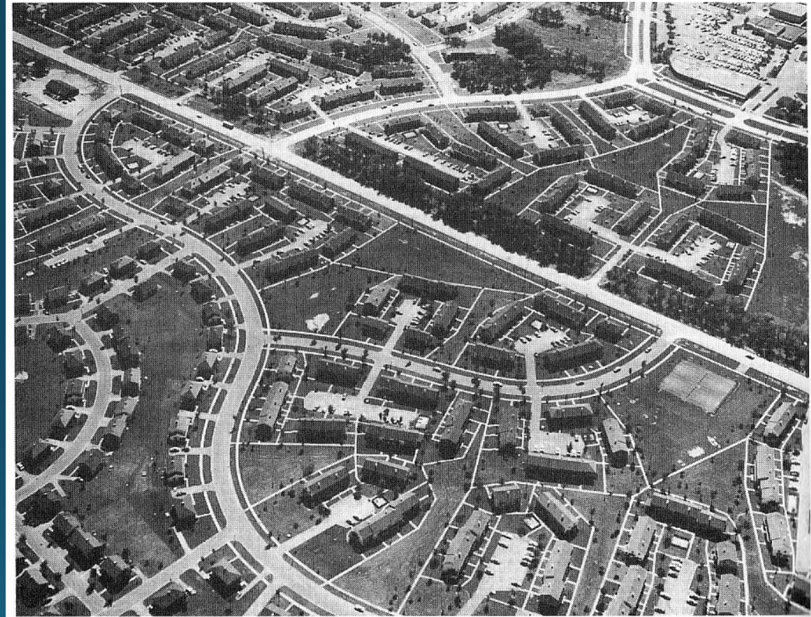
Fig. 30. The “superblock” concept of apartment development is obvious in this view of the community under construction in the early 1950s. Source: courtesy of Park Forest Public Library.
