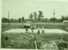
8 AM Site and wall panels arrive at site.
