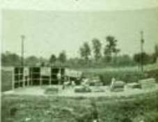
9:55 AM Wall panels are raised in place.
