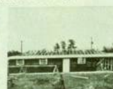
1:26 PM Sheathing is nailed to studs.
