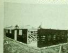
10:10 AM Roof trusses are set on walls.
