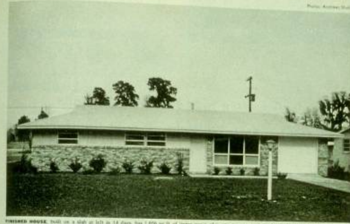
FINISHED HOUSE, built on a slab at left in 14 days, has 1,076 sq ft of living space plus one-car garage (see details, this p. 107).
